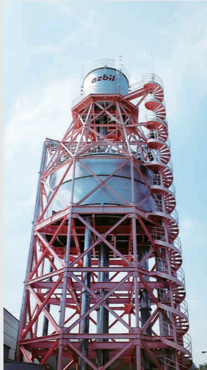
Elevated water tank for calibration
