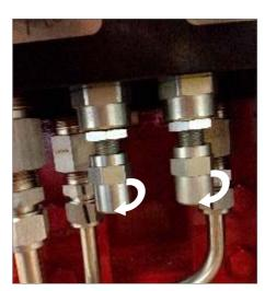
Fig 10.4 Flow regulator cap removal
