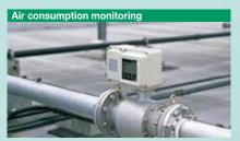
A mass flow meter is necessary to measure the actual load and air consumption of a compressor. This product can precisely measure the flow with no need for adjustment in temperature and pressure.
