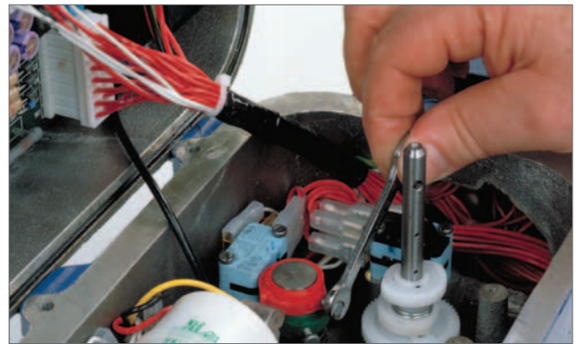
Torque switch setting
