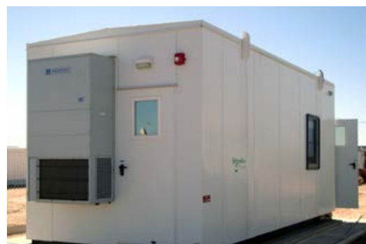
Fully equipped power house with switchgear, PLCs, HVAC, and fire and gas system to control and operate two MP1-380 units in Argentina
