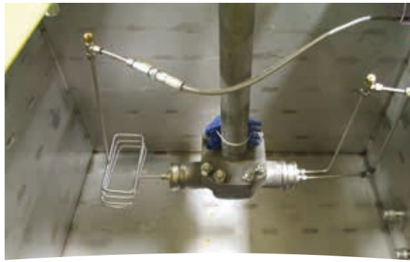
2" McCANNA CryoSeal test preparation
