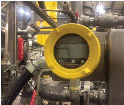
One Series Safety Transmitters are shown mounted on Gas Processing Units that provide SIL 2 SIF pressure monitoring for natural gas separation skids
