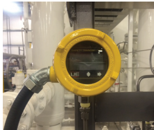
One Series Safety Transmitters are shown mounted on Gas Processing Units that provide SIL 2 SIF pressure monitoring for natural gas separation skids
